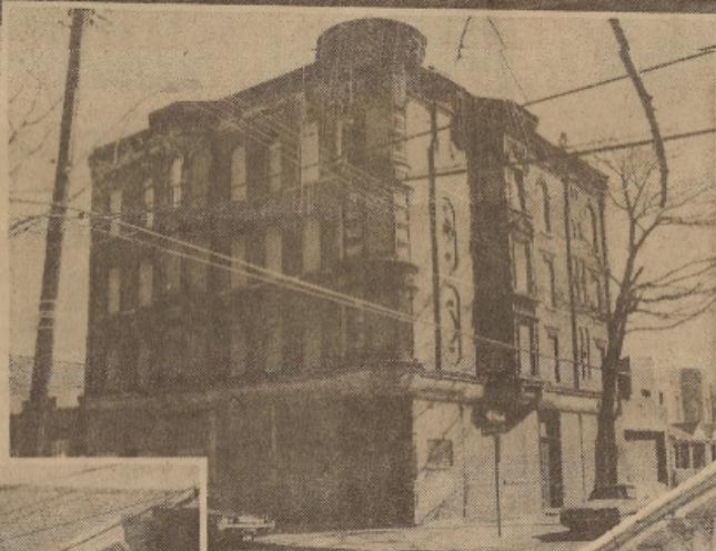
Wyckoff Building, 93-02 95th Ave., is another landmark of old Woodhaven Village. It is considered a figurehead of old village.
